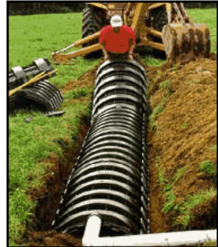
FIGURE 1 LEACHING CHAMBER
