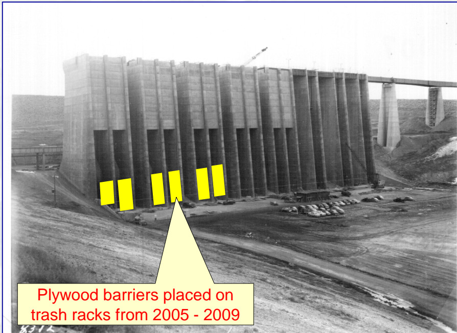
Garrison Dam 10 Dec. 1952
