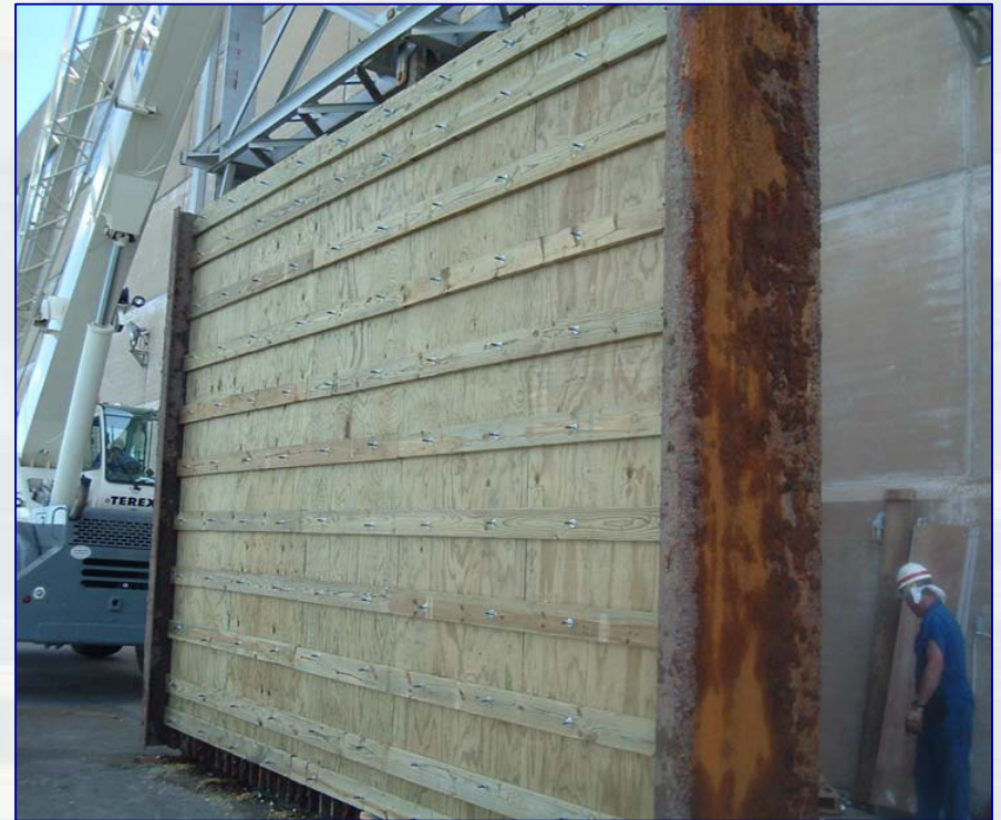
Trash Rack Section with Plywood Installed
