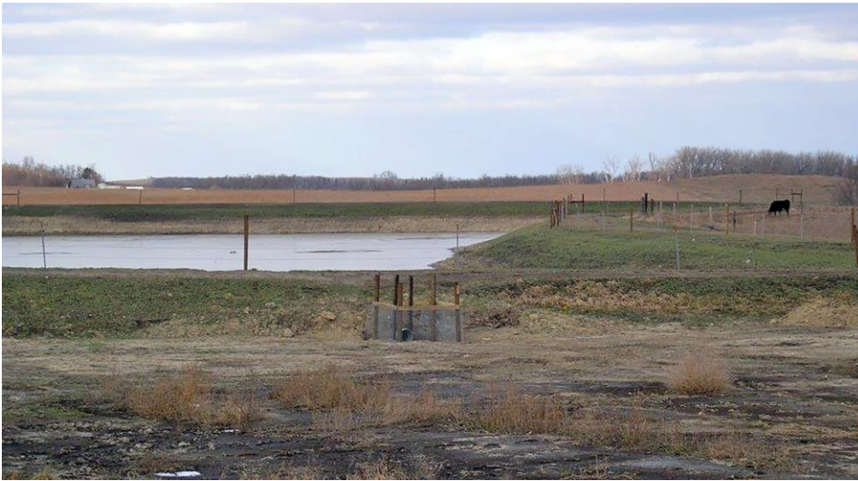
Livestock waste management containment pond and fencing.
