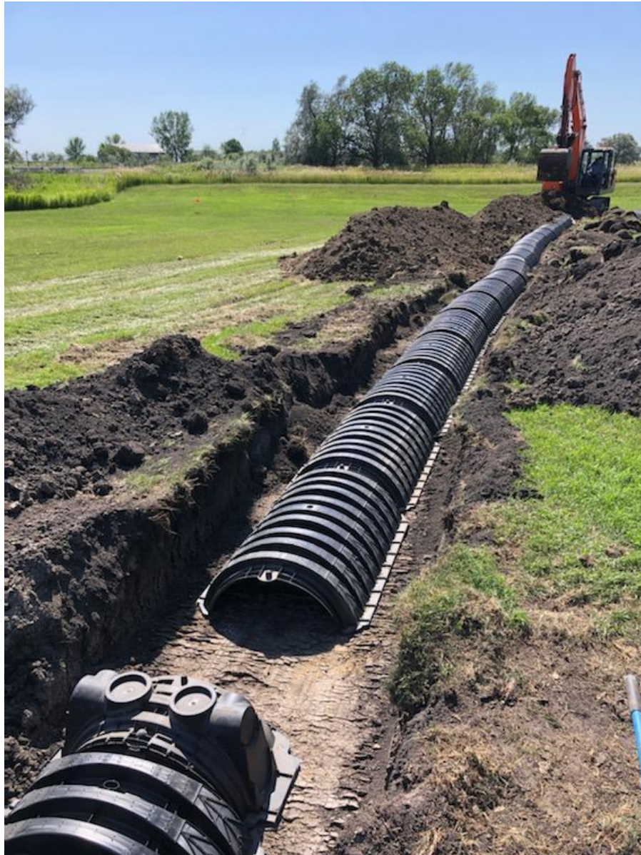
Fig.7. Installation of a new septic system along the English Coulee.
