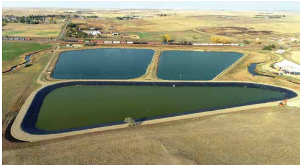
Hettinger, ND, waste stabilization ponds. Image source: broszengineering.com.
