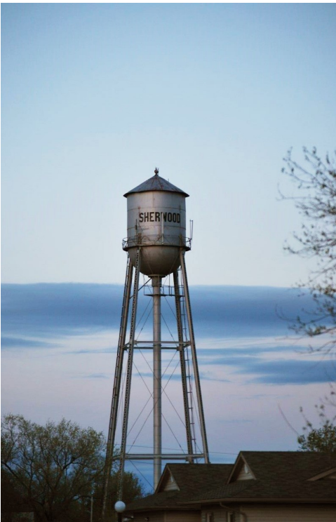
A water tower providing the town of Sherwood with drinking water. (ND Tourism)
