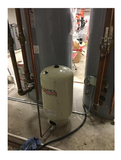
Wrong expansion tank for storage water heaters, bigger than 5 gallons... must be ASME
