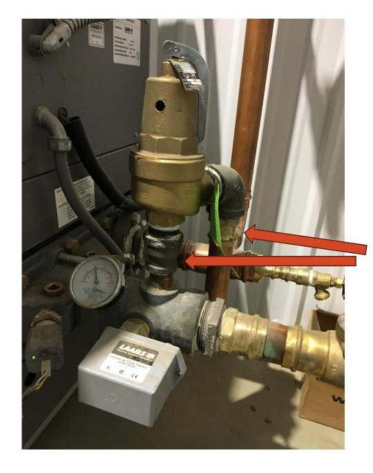
Reduced safety relief valve inlet and outlet...
