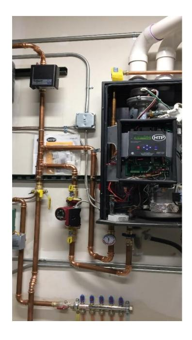
Low water fuel cutoff in the secondary piping after coming out the bottom of the boiler
