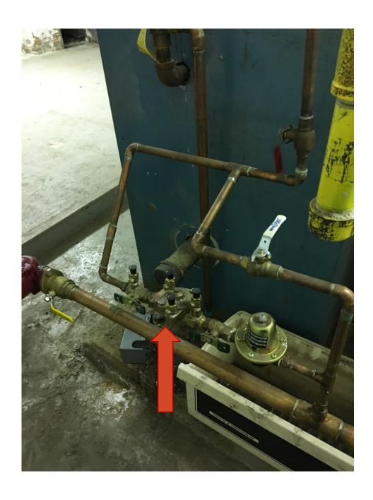
Bypass just the feed water regulator, not the backflow preventer
