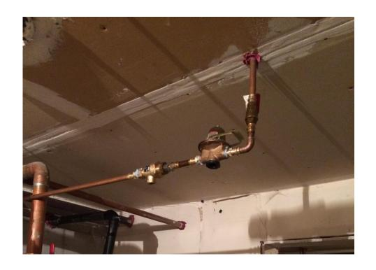
Feed line troubles – not RPZ, on low side, no bypass and no feed stop valve
