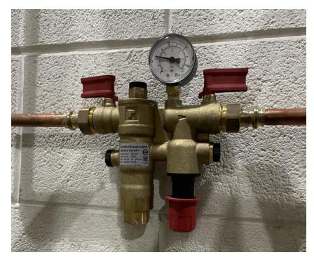
Feed trouble – cannot install bypass for regulator and not RPZ – not for commercial install
