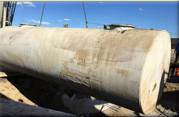
Removing an underground storage tank
