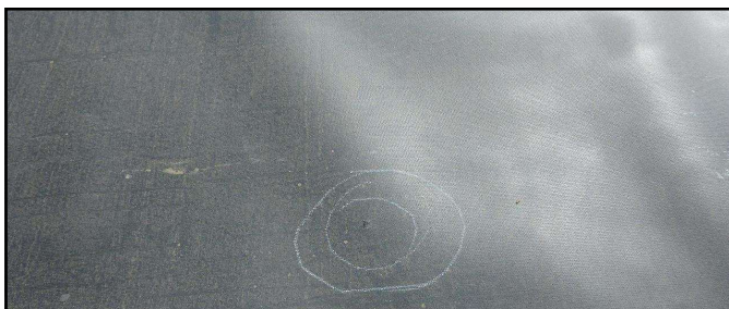
LINER Hole identified
