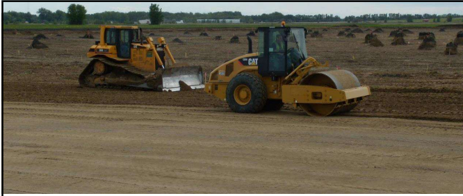
LINER COMPACTION Clay Material
