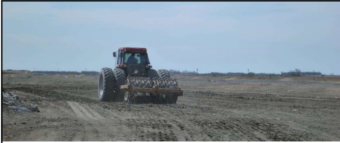
LINER COMPACTION Clay Material
