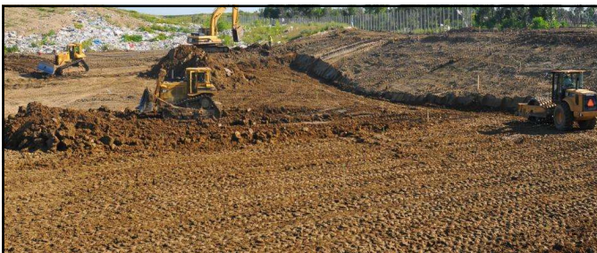
LINER COMPACTION Clay Material
