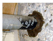
BROWN CAULK AT PIPE PENETRATION
