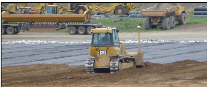
DRAINAGE LAYER Spreading
