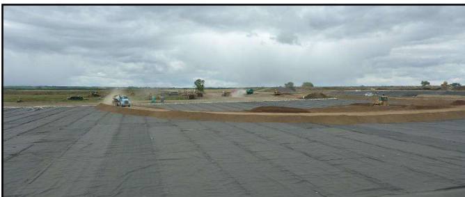
DRAINAGE LAYER Truck Haul Road
