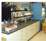
ASBESTOS CEMENT COUNTER TOP (STAUFER 8)
