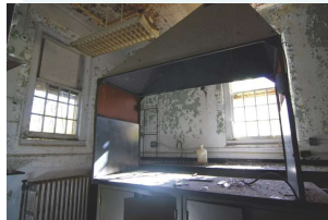
ASBESTOS CEMENT COUNTER TOP (STAUFER 8)
