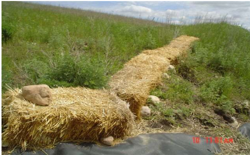
Straw Bales used for Final Cover Erosion Control
