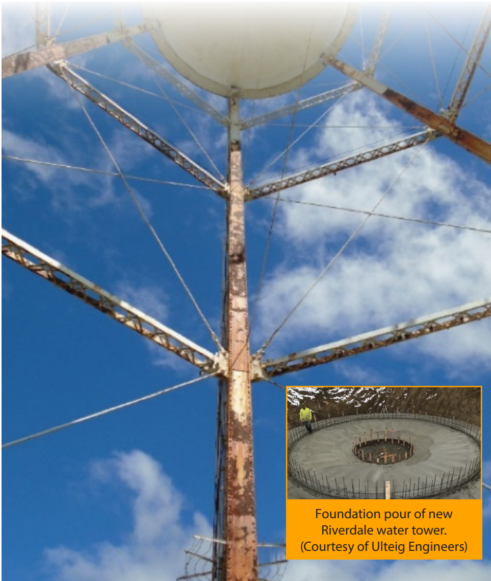
Corroded structure of existing water tower. (Courtesy of Ulteig Engineers)
