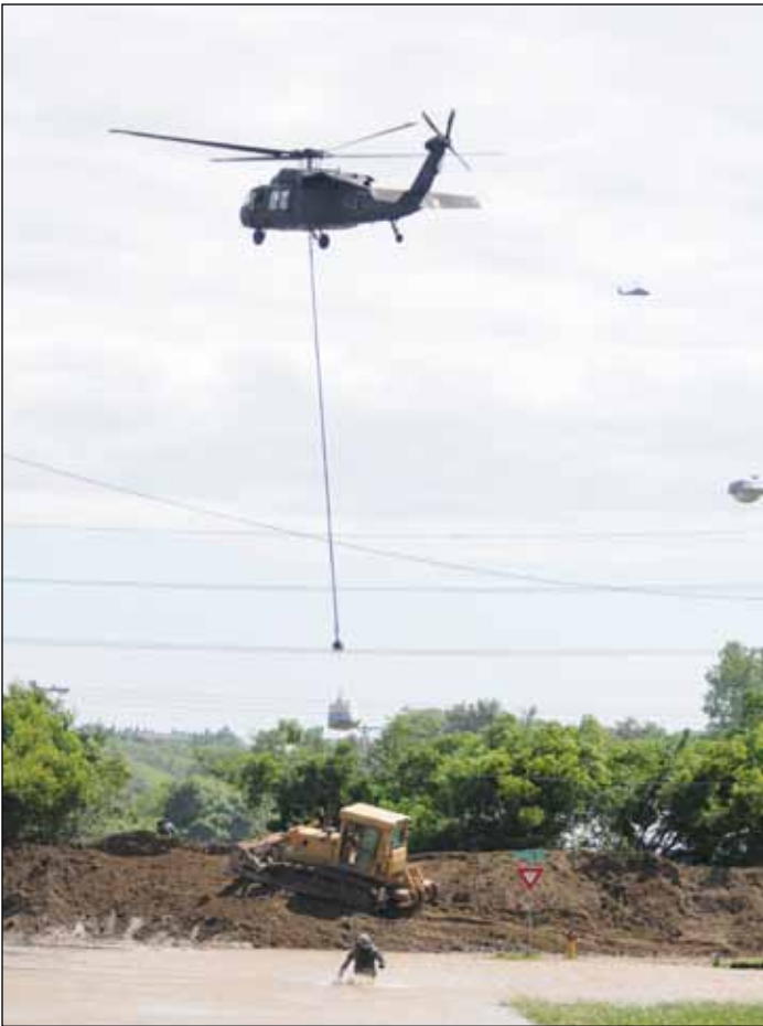
The North Dakota National Guard assisted the city of Minot greatly. On June 24, 2011, the Guard used a UH-60 Black Hawk helicopter to quickly reinforce a flood levee at 13th Street and Railway Avenue with a 1-ton sandbag. (photo by Senior Master Sgt. David H. Lipp)
