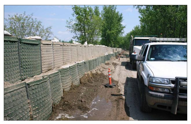
As the forecasted river stage continued to climb, the initial HESCO<sup>TM</sup> barrier along Riverwood Drive was bolstered by adding another row of barriers and stacking a third row on top. Note the seepage occurring in the foreground. The highest river stage eventually resulted in about 4 feet of water against these barriers. Photo by Mel Bullinger, city of Bismarck, June 3, 2011.
