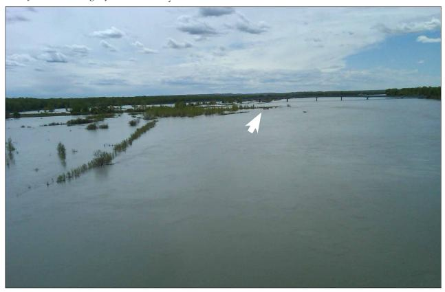
View of Bismarck's horizontal collector well construction site and access road in late May 2011. The Missouri River stage was 15.77 feet. Eventually in June it exceeded 19 feet, resulting in a river depth approximately 13 feet higher than in the prior photo. Photo taken from the same vantage point as above. Photo by Ken Weber, AE<sub>2</sub>S.
