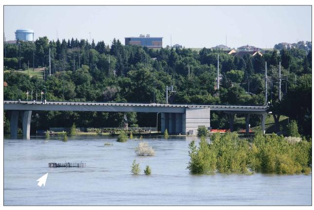
The rising Missouri River inundates all but the reinforcing steel (arrow) at the very top of the existing caisson for the new horizontal collector well, currently under construction for Bismarck's water treatment plant. Photo by Mel Bullinger, city of Bismarck, July 4, 2011.
