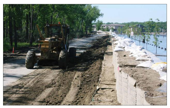
A city of Bismarck grader blades a wedge of clay material against the HESCO<sup>TM</sup> barrier dike along Riverwood Drive in Bismarck. Note the flooded parking lot and marina on the river side of the dike. Photo by Mel Bullinger, city of Bismarck, June 3, 2011.
