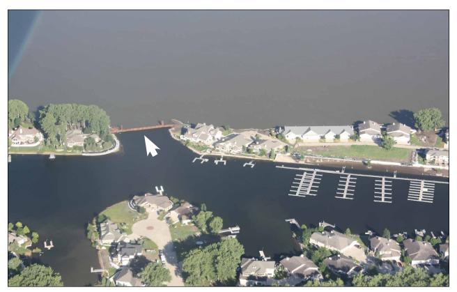
This sheet piling dam (arrow) was privately built to control the water entering the Southport residential area. Water was then pumped out of the bay to lessen the impact of the flood. Photo by Mel Bullinger, city of Bismarck, July 11, 2011.
