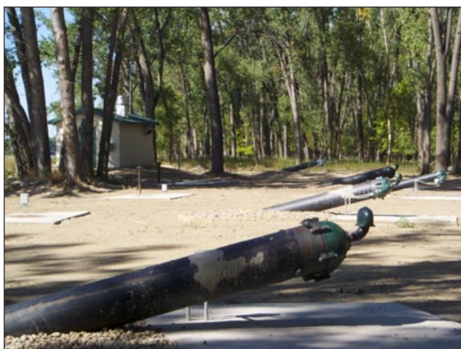
Completed angle wells and pump control building
