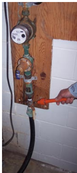
Listening for leak noise on a service line.
