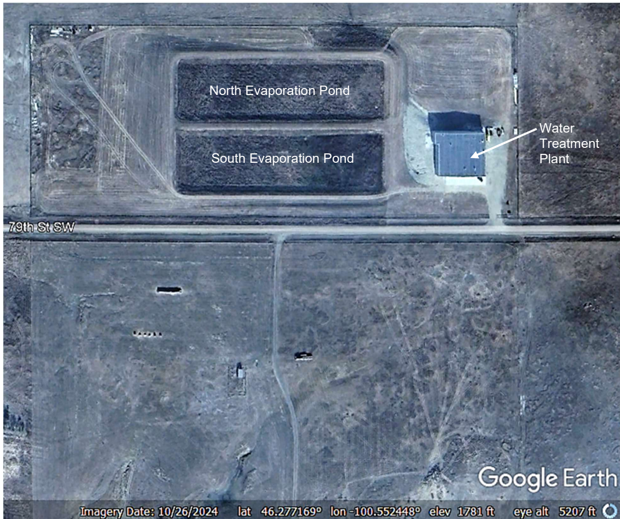
Figure 2: Google Earth imagery (dated 10/26/2024) for South Central Regional Water District – Emmons County Water Treatment Plant and Evaporation Ponds.
