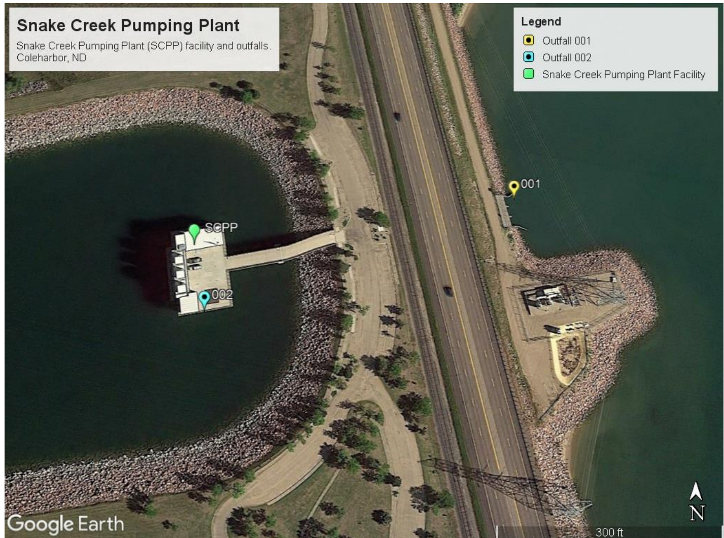
Figure 1. Aerial Photograph of Snake Creek Pumping Plant (Google Earth Pro, Map Generated on 03/27/2023).
