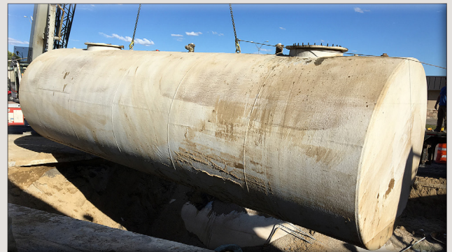
Removing an underground storage tank
