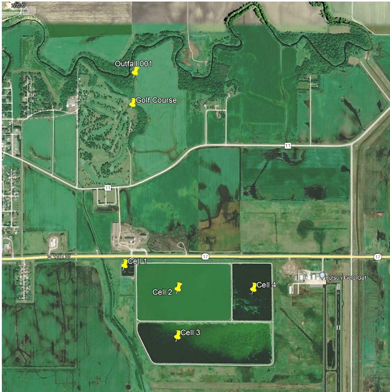
Figure 1 – Grafton Wastewater Treatment Facility Overview (Google Earth 7/24/2020)
